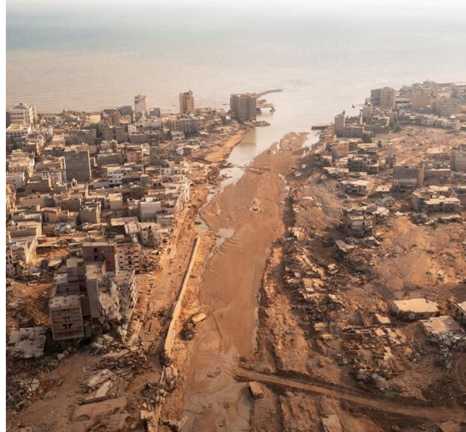
Flooding in Derna, Libya.
