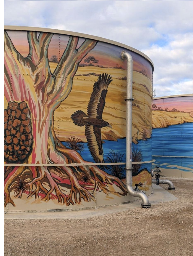
Remote water tank system.
