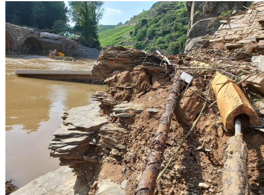
Destroyed Infrastructure in Ahrtal/Germany
