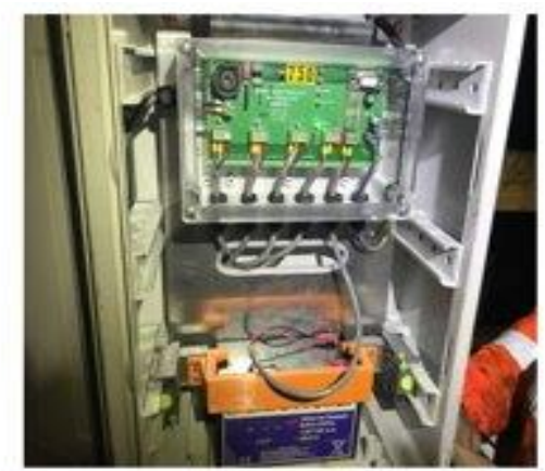
Bridge of Orchy RDN Wired Satellite Telemetry
