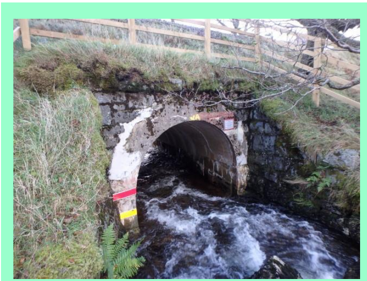
INITIAL TRIAL SITE: Underbridge 310/184A West Highland Line WHL 55m+0270yds
