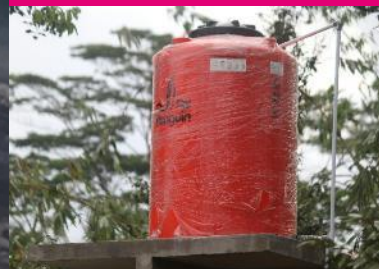
Fill Level Monitoring
