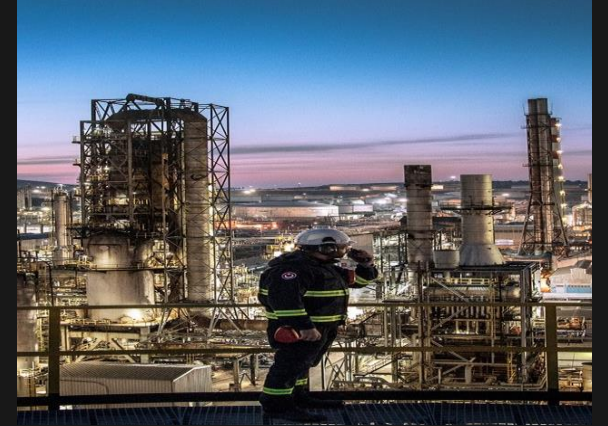
Izmit, Tupras Refinery Turkey
