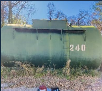
Water tank levels monitoring
