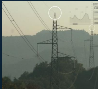
Power line monitoring
